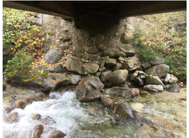
Left Bank Abutment when facing downstream
