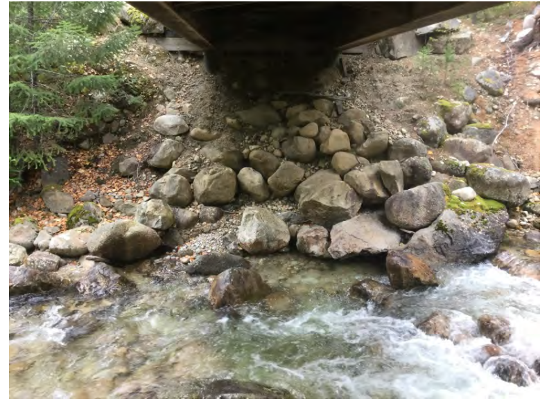
Right Bank Abutment when facing downstream
